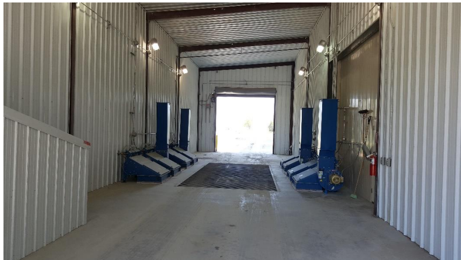
Figure 4.5. Drive-through receiving pit with heavy duty grate and dust suppression and control system. Note cleaning tools including brooms and shuffles hanging on the wall for easy access to cleaning up the receiving pit area after trucks have been unloaded.
