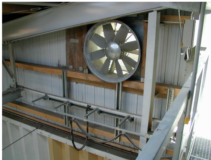
Figure 4.17. High airflow, low electric power exhaust fan venting headspace air from a flat storage building.
