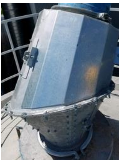
Figure 4.6. Example of a cushion box that reduces grain velocity as grain flow comes in contacts with the “cushion” as a result of grain contacting grain instead of metal surfaces.
