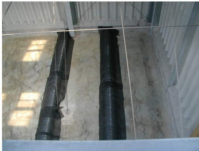
Figure 4.18. Semi-permanent aeration system showing half-round perforated on-floor ducts to aerate grain in a flat storage building before it is filled
